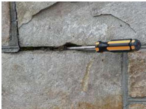
The front elevation upper area mortar joints are cracked and filled with wet, deteriorated mortar.
